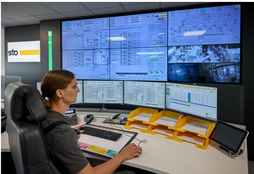
The control center at Sto.
