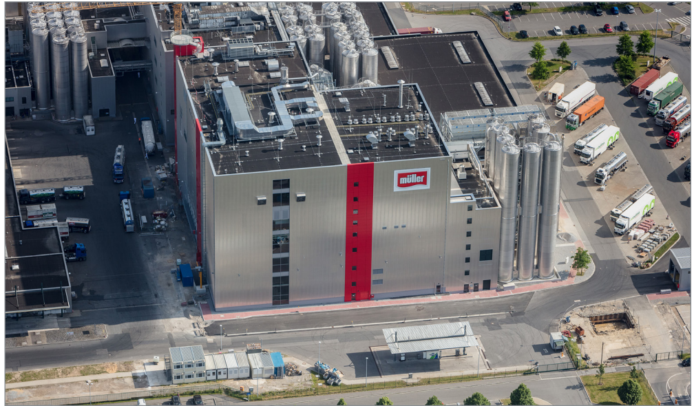
The 'Molke 5' building
